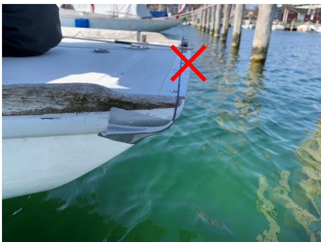
Intersection between the deck and the transom seen athwartships
