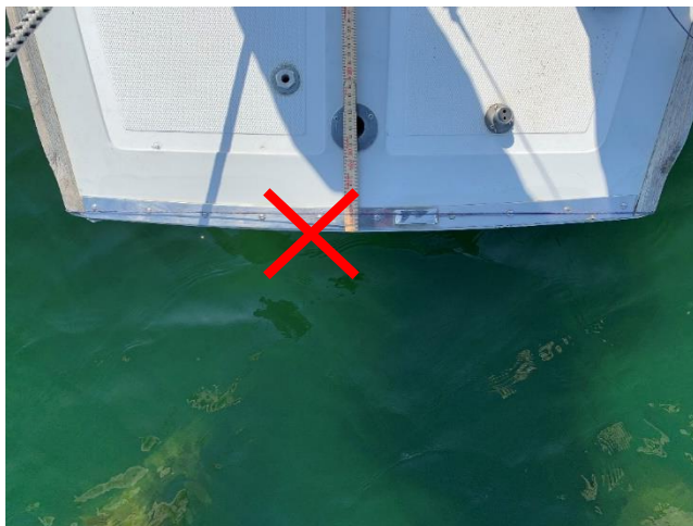
Intersection between the deck and the transom seen from above
